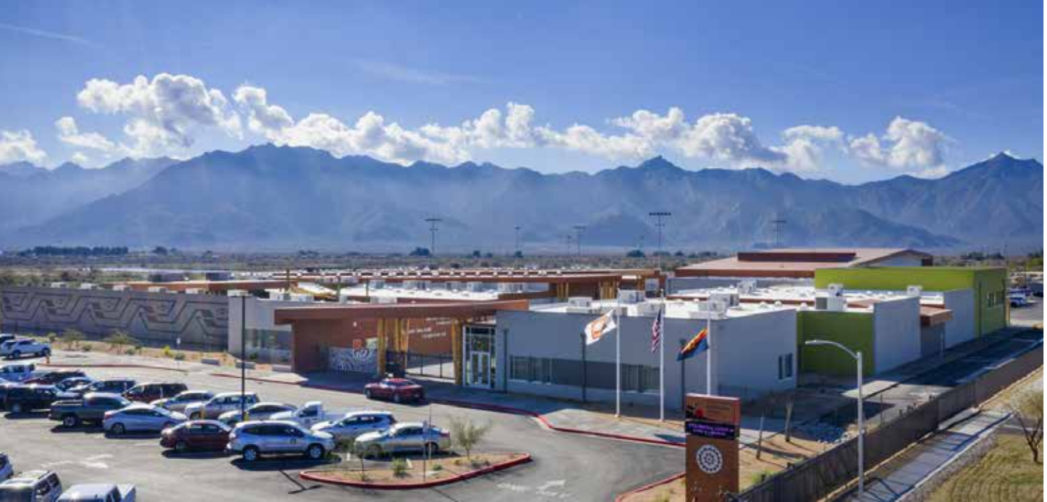
The lease for the Gila Crossing Community School was executed as part of the Department of the Interior's section 105(l) leasing program contained in the Indian Self-Determination and Education Assistance Act (ISDEAA).
