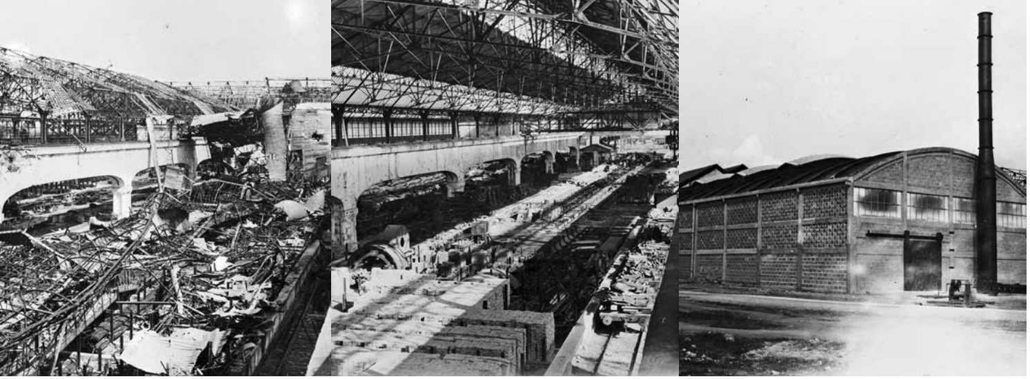
Left: A French steel plant in 1945. Center: The steel plant was almost back to prewar production level in 1948, thanks to reconstruction and raw material supplies under the Marshall Plan. Right: The same plant newly reconstructed in 1948.
