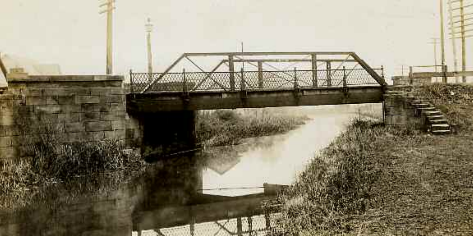
National Road bridge over Ohio & Erie Canal at Hebron, 1910.
