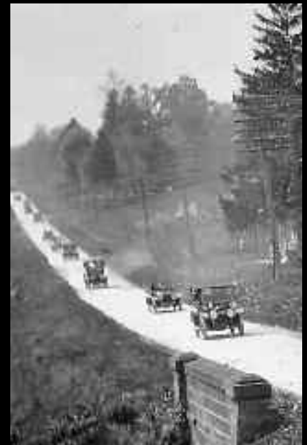
Caravan on new concrete Road west of Zanesville, November, 1916.
