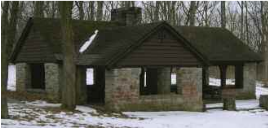
This picnic shelter at Taylorsville MetroPark was constructed by the Civilian Conservation Corps (CCC) in 1938 and restored by the CCC in 1989.
